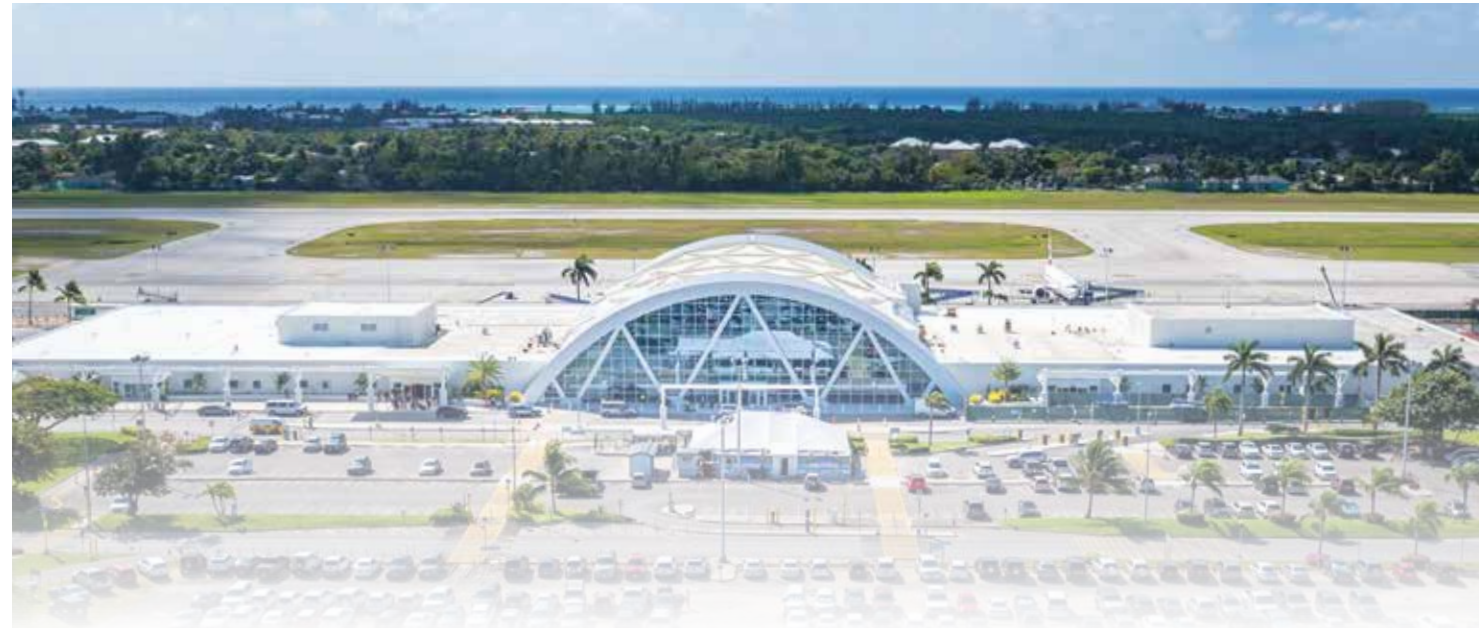
Owen Roberts International Airport expansion
